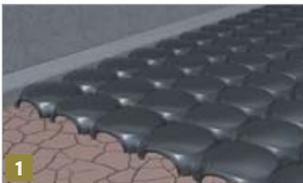
1 Lay the interlocking male/female formworks directly on the dry ground, from left to right and top to bottom, ensuring that the arrow marked on the Coffrargile formwork is facing up.
