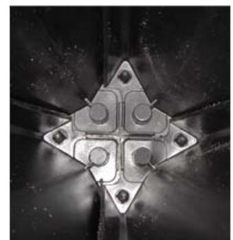
Detailed view of the male-female system linking phase - note the perfect seal of the feet.
