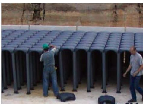
In comparison to collection tanks, dispersion tanks are not perfectly waterproof but permit the gradual release of the rainwater to the water bed through slits in the walls or draining bottom.
