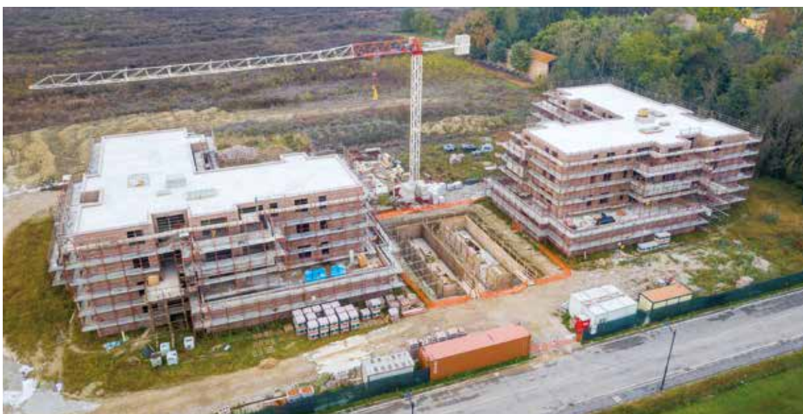
Intervento Social Housing 40 alloggi a Molinella (BO) - 2020
